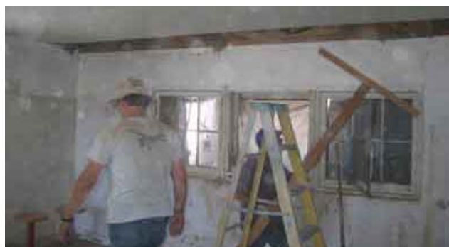
Sheet rock being installed.
